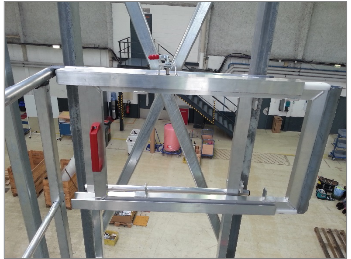
Sliding guardrail to be near optimum to the wing
